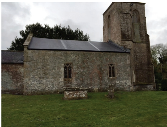
All Saints' with the new rubberoid roof
